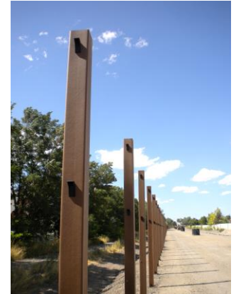
Brackets are attached to the Composite Posts at Rail Points
