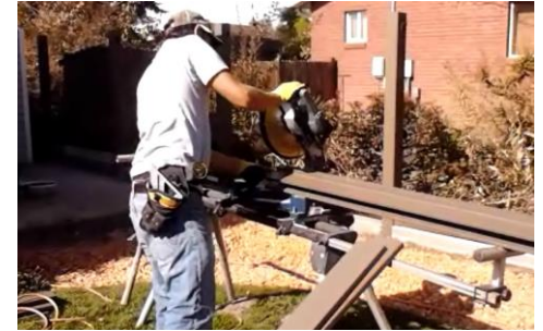
Trex materials are cut with miter and circular saws (non-ferrous blade is used for aluminum rails)
