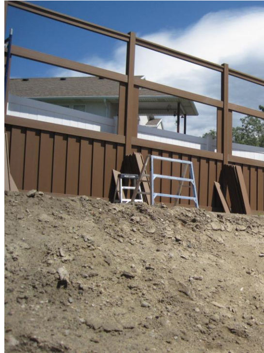
Fence is built from the bottom up using intermediate aluminum rails with composite covers
