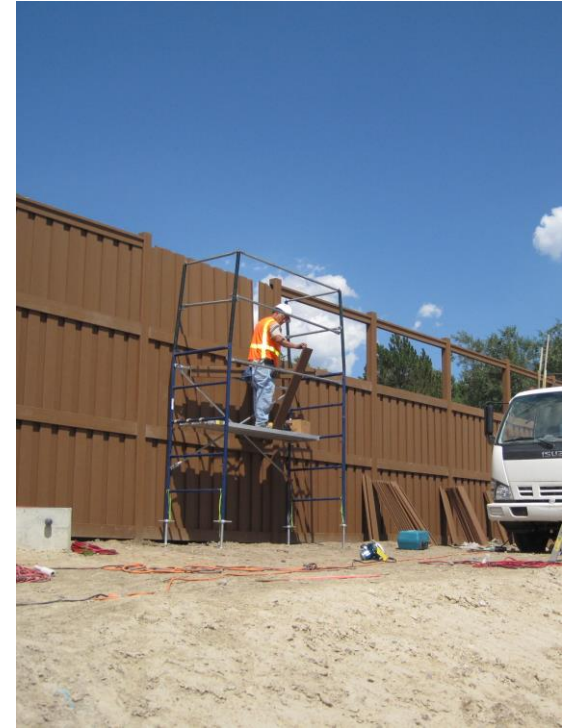
Pickets are interlocked and the top rail is placed over the pickets to ensure the fence is secure
