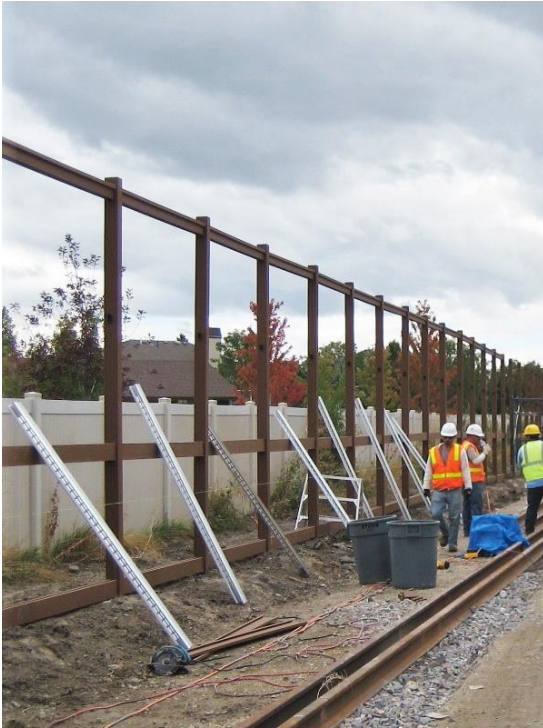
Rails are placed temporarily for accurate measurements
