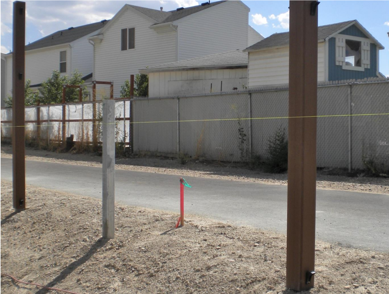
3.5"x3.5"x3/16" Galvanized Steel Post Stiffeners are set in concrete
