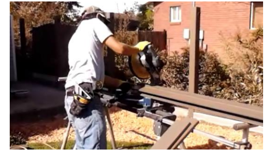
Trex materials are cut with miter and circular saws (non-ferrous blade is used for aluminum rails)
