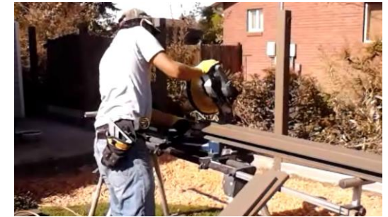
Trex materials are cut with miter and circular saws (non-ferrous blade is used for aluminum rails)
