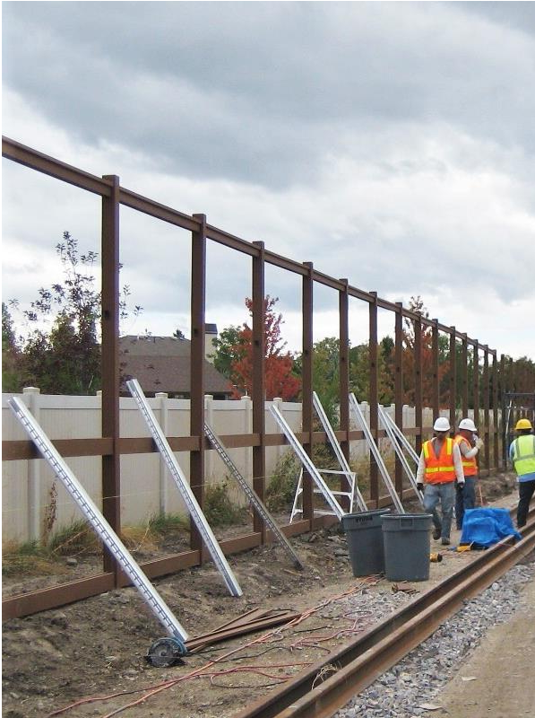
Rails are placed temporarily for accurate measurements
